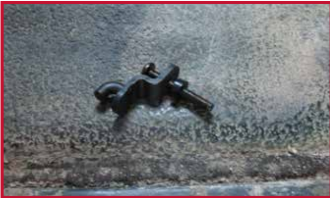
Figure 7 - Hook and Spacer Assembly
